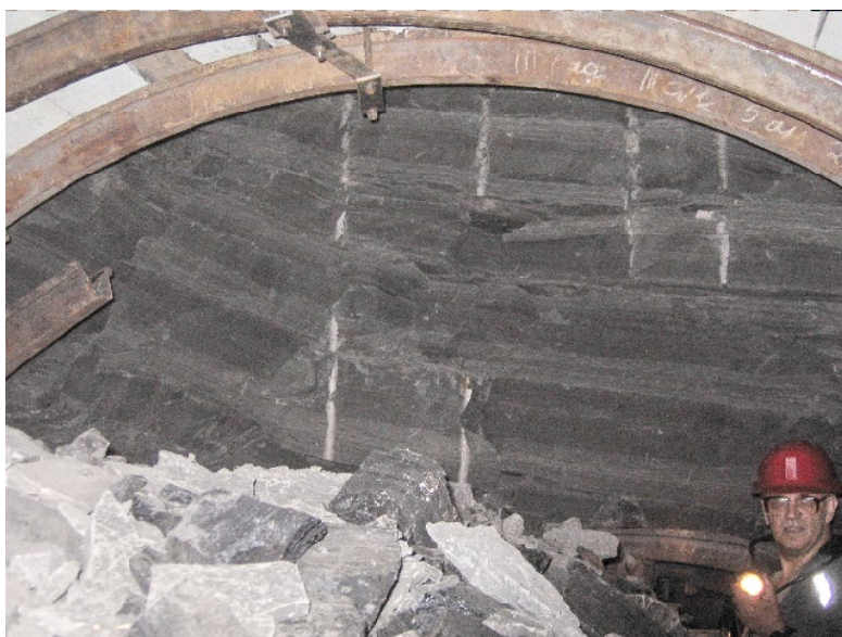
Figure 2 – Photo of the rock-bolts block, which was taken during the re-supporting of the emergency region of the 351 roadway
